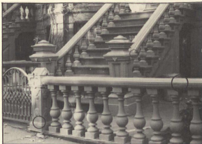
Well-maintained cast iron; all repairs done by owners as soon as problems appeared. Details below.
