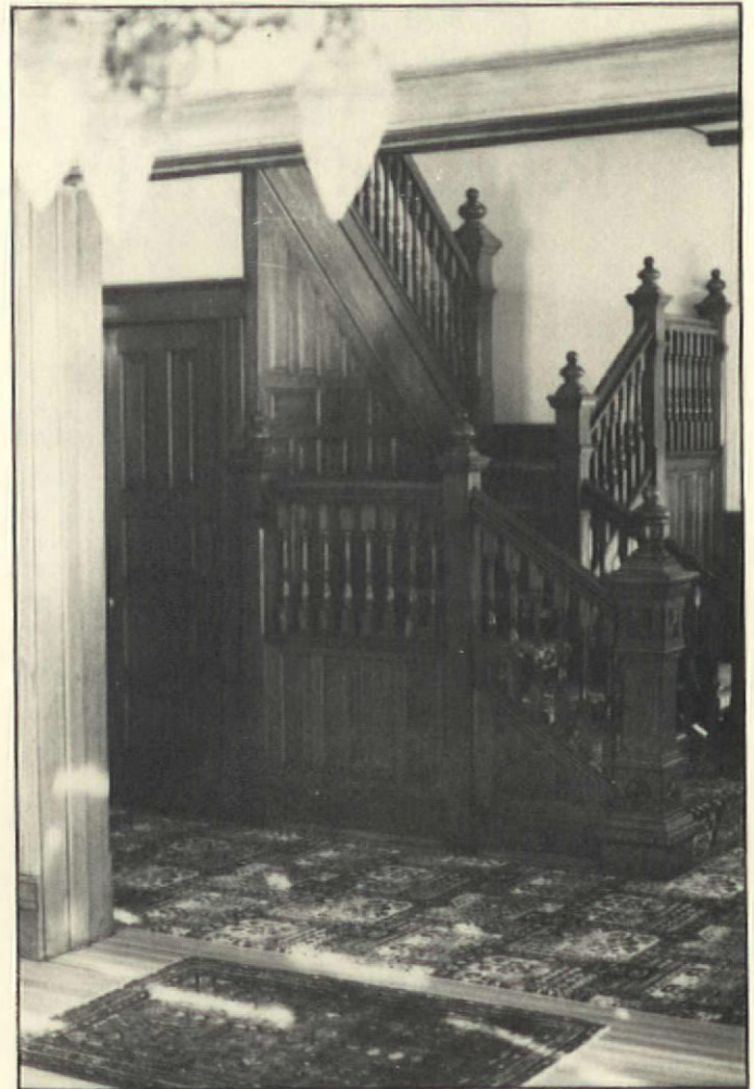
Entry halls with elaborate wood staircases and turned spindles are a common feature in Queen Anne style houses.
