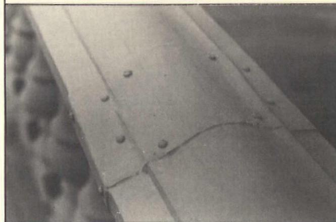
Closeups belie small size of these sheet-metal patches, held by screws and caulk, done 30 years ago.
