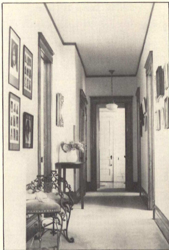
Upstairs hall is papered with a vinyl that looks like raw silk. Baseboard, moulding and door frames have been stripped.
