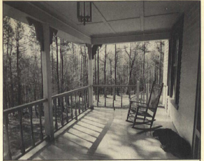
Second floor porch shows the darker paint (Charleston blue) accents on the porch brackets, balustrades, door and window frames contrasting with the sand-colored body paint.
