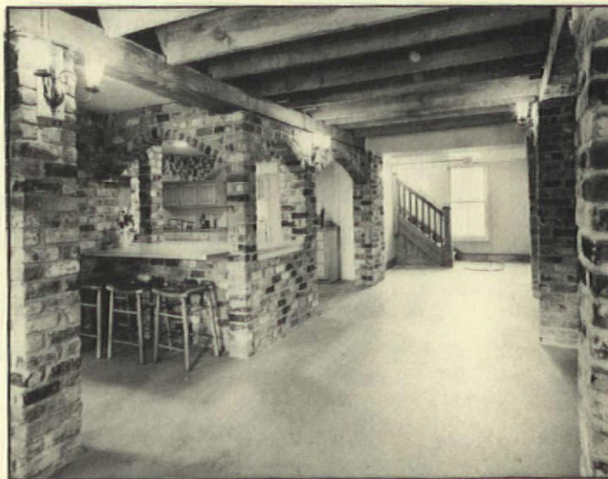
Looking through the arches to the New Orleans kitchen. Note the handhewn pine beams (floor sills).
