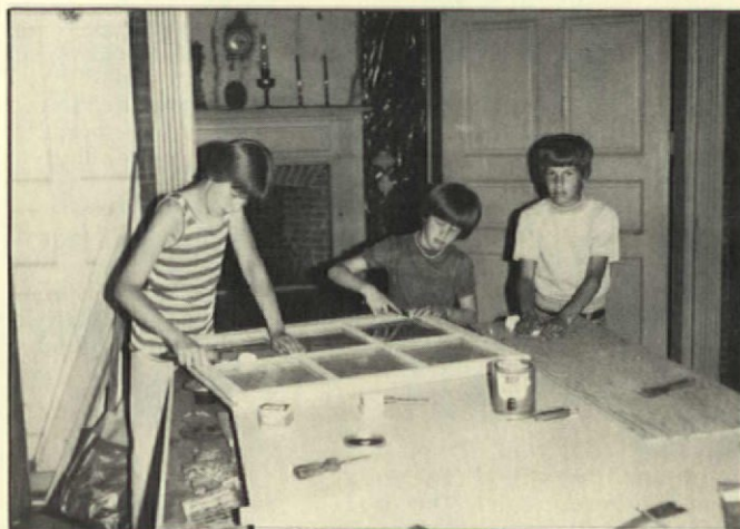
The children are putting the old glass from the rotten sash into the new sash.
