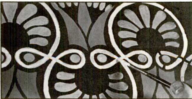
6. Gaps left in pattern by the ties are filled in by hand. Since paint in stencil pattern is thin and partially translucent, it takes some practice to get the painted-in areas to blend nicely.
