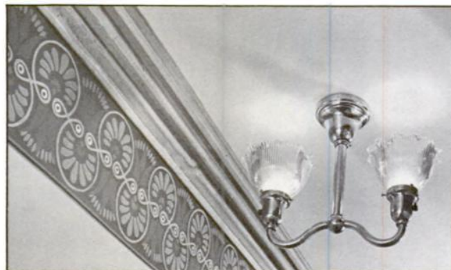
The varied tones on the glazed moulding were produced by leaving a heavier residue of glaze on the receding portions.
