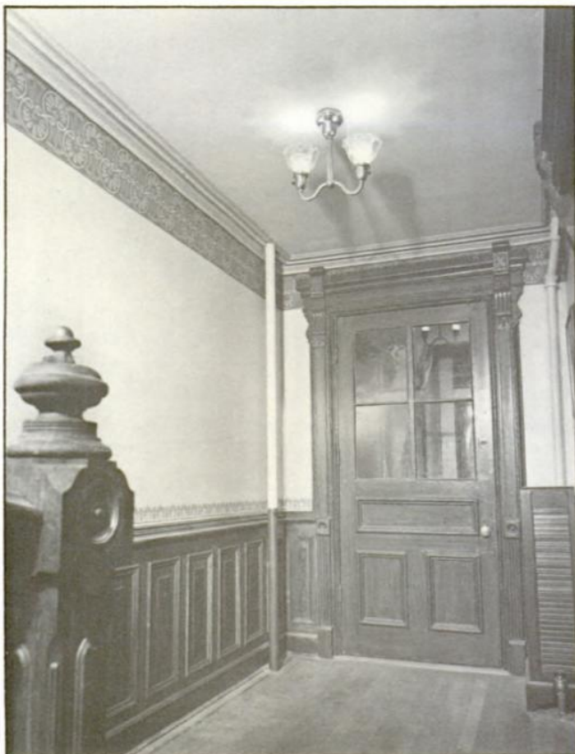
This view of the hall shows the duplicated walnut wainscoting on the left. The rest of the woodwork, including the radiator enclosure, is grained.
