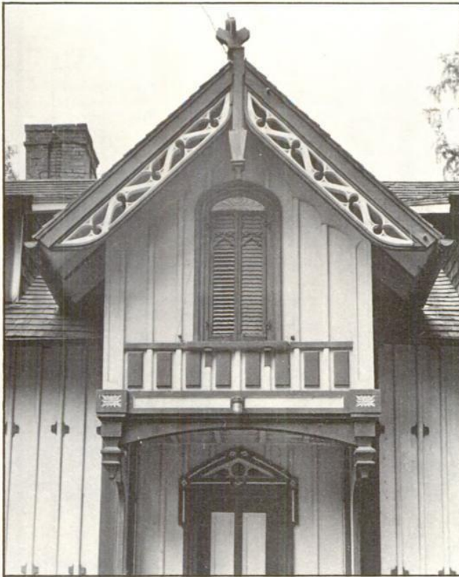
This section of a Gothic Revival cottage designed by Andrew Jackson Downing is a good example of the Victorian manner of painting houses. Architectural decoration is emphasized by the use of light and dark paint. (Photo courtesy of the Dutchess County Planning Commission)
