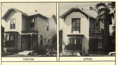
Exterior restoration included ripping off the asbestos shingles and repainting, installing finials at roof peaks, creating a widow's walk atop the house, re-creating much gingerbread trim, and replacing the door and railing for the small second-floor porch over the front door.
