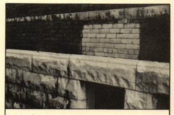
Sometimes paint isn't the problem...just years of accumulated dirt and grime. This test patch shows how a chemical cleaner will quickly restore the original look.
