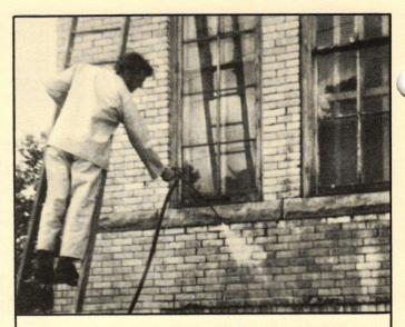
Thorough flushing of the brick cleaner requires a high-pressue (300-500 psi.) hose to remove all surface dirt. This equipment can be rented.
