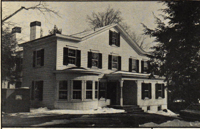
Rear of house shows a variety of additions made to the structure during the 19th century. Victorian bay window, with decorative shingling beneath cornice, gives distinctive shape to the "Oval Room." It was built sometime between 1878 and 1900.
