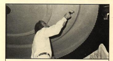
Jim Geraghty is priming the ceiling. The stencils have already been made and are ready to be applied. The tan paint is a few shades darker than the final coat will be—the way to prime when painting with colored paint.
