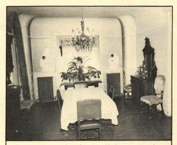
Much work remains in the dining room. The wainscotting is oak—and heavily painted. A heavy plaster moulding had been removed from the ceiling perimeter and plans are to replace it. Wiring for the sconces was added in the 1930's, walled over in the 1950's and uncovered in the 1970's.
