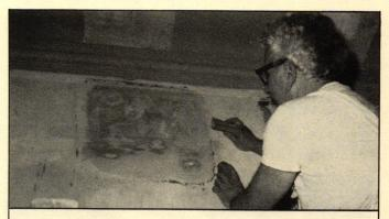
Howard Zucker, of Rambusch, has uncovered enough of the lotus flower design in the frieze to make a stencil. After removing 5 or 6 layers of paint with paint remover, until a trace of pattern appears, he then sands with very fine wet and dry sandpaper.
