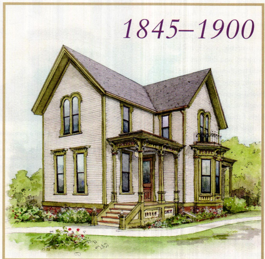
A familiar cross-gabled house dressed in Italianate details: note the tall windows with heavy hoodmolds and round tops, the fancy wooden brackets, three-sided bay, and ornamental ironwork.
