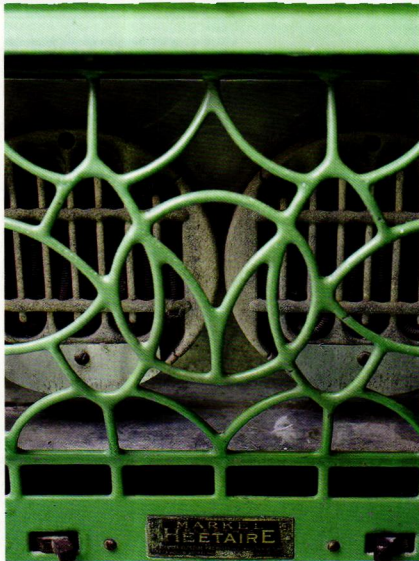
The built-in enameled electric fan/heater combo made by Markel Electric features an attractive grate with a stylized M, presumably for Markel.
