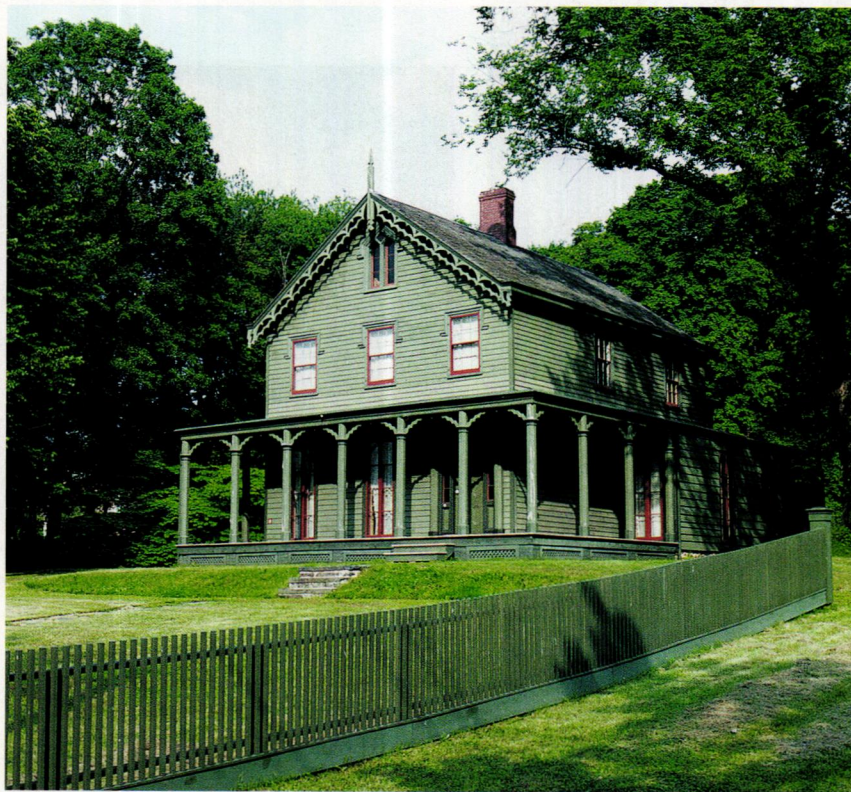
An 1855 parsonage at Historic Richmond Town in Staten Island, New York, originally had a cream body and Venetian red trim. Around 1870, when the Carpenter Gothic gable ornament was added, exterior colors were changed to this more saturated, late Victorian scheme featuring a green body.
