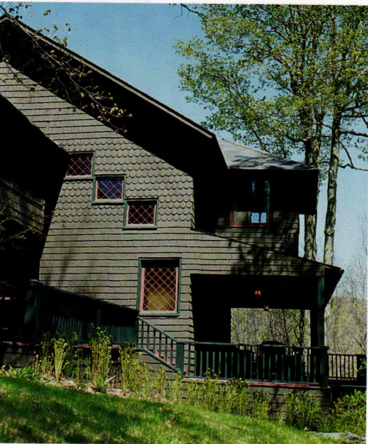
ABOVE: The house was built in 1893 by Miss Adelaide Hazelhurst and is similar to several other Onteora cottages designed by Dunham Wheeler. RIGHT: The generous front porch offers views over the Catskills.
