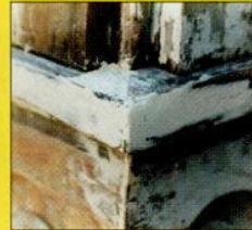
Consolidation and rebuilding of rotten windowsill with LiquidWood and WoodEpoX .
