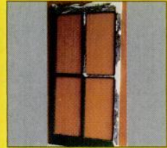
Antique window sash is salvaged, consolidated with LiquidWood and rebuilt with WoodEpoX .
