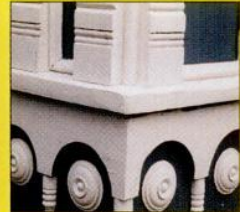
Consolidation and rebuilding of rotten windowsill with LiquidWood and WoodEpoX .
