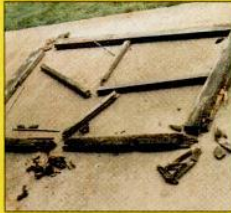
Antique window sash is salvaged, consolidated with LiquidWood and rebuilt with WoodEpoX .
