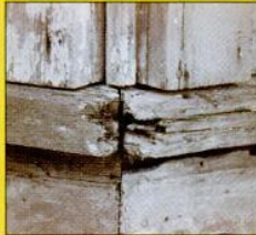
Consolidation and rebuilding of rotten windowsill with LiquidWood and WoodEpoX .
