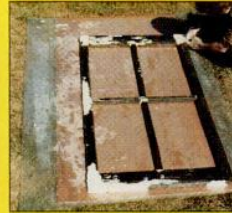
Antique window sash is salvaged, consolidated with LiquidWood and rebuilt with WoodEpoX .
