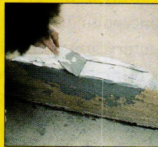
AboWeld 55-1 , is much stronger than concrete and shapes without forms on steps and difficult surfaces.
