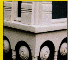
Consolidation and rebuilding of rotten windowsill with LiquidWood and WoodEpoxy .
