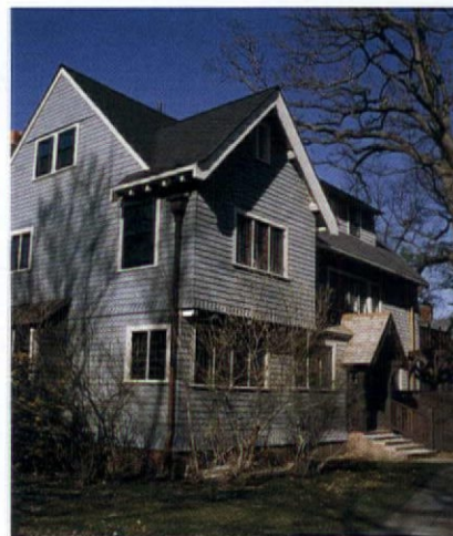
ABOVE: An unassuming façade gives no hint that the house was rebuilt two years ago. LEFT: A bank of windows overlooks a leafy back yard. Cabinets in the new kitchen are patterned on those in the original butler's pantry.
