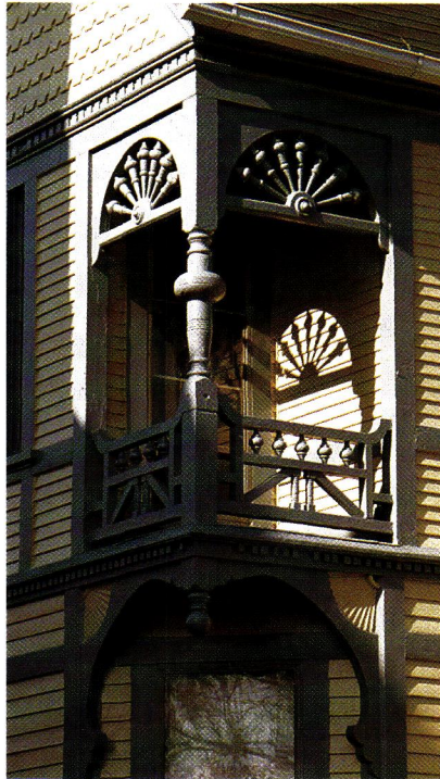
Even a tiny porch is ornamented with ball-and-spindlework fanlights, ornate railings, and an unusual turned post.
