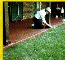
Rotted & infested base of a loadbearing column is completely sawed off and replaced with WoodEpoxy .
