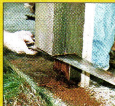
Rotted & infested base of a loadbearing column is completely sawed off and replaced with WoodEpoxy .
