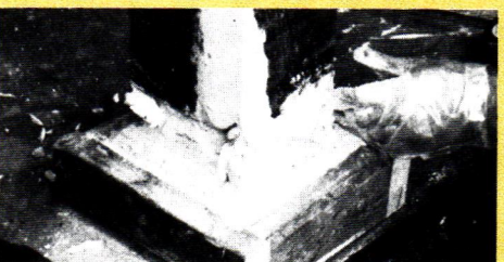
...were completely sawed off and replaced with...
