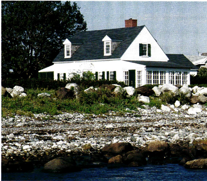
The porches at either end were added early in the 20th century, but the house's footprint is the same as it probably has been for two hundred years. RIGHT: From a porch, a view of the harbor.
