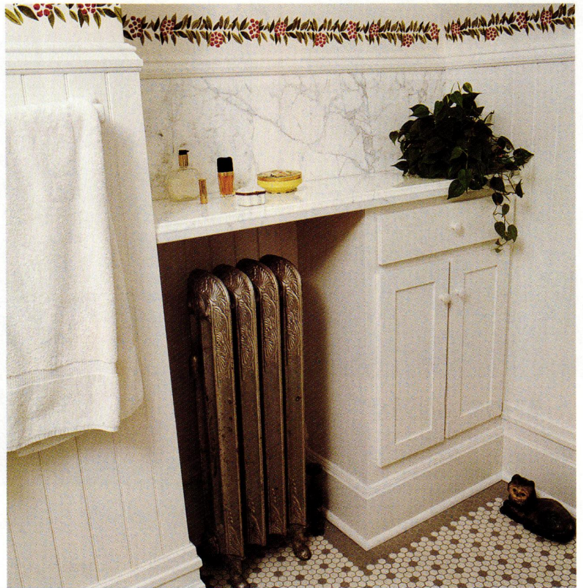
LEFT: Paneling of the 1960s suited the dark and dispiriting floor and cabinet. ABOVE: Elmhurst, Illinois, craftsman John Hammond installed beadboard, marble, tile, and a baseboard that recall turn-of-the-century conventions.
