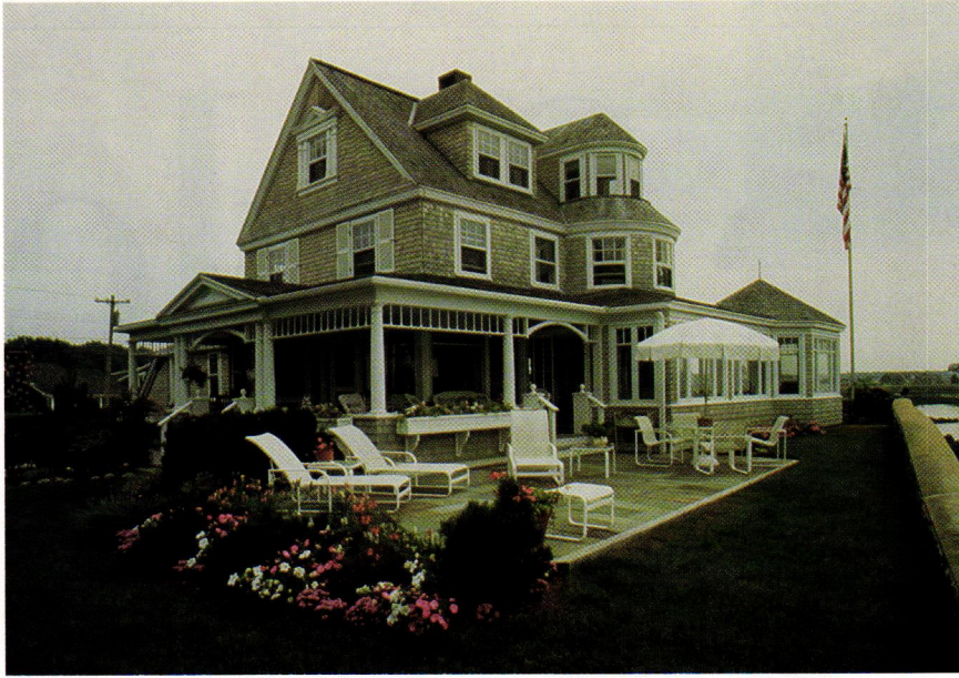
This c.1884 house in Kennebunk, Maine, was recently rescued from aluminum siding and rot. Porches are rebuilt.
