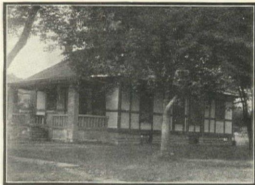
Bungalow designed by White & Sons, Architects, Clarion, Iowa, sided with Asbestos Building Lumber
