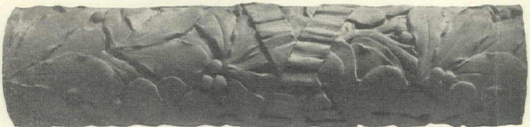
Concrete Ornament Applied to Facade.
