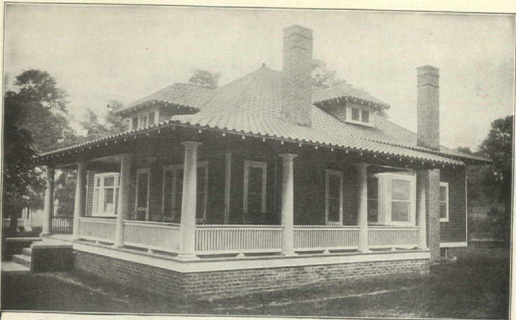
Bungalow Roofed with Edwards Metal Spanish Tile. W. C. Burrell, Atlantic Highlands, N. J., Owner Conover E. White, Sheet Metal Contractor
