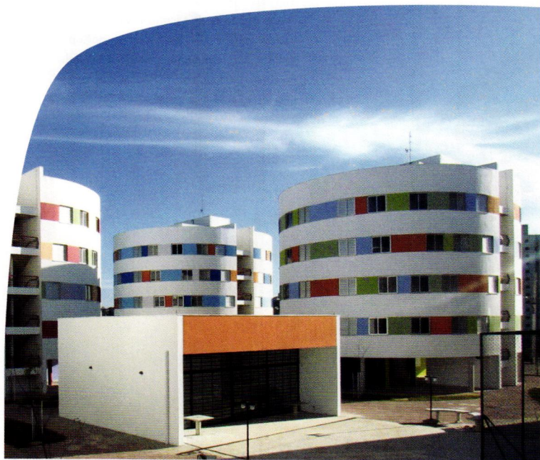
The "Redondinhos," government-funded residential buildings in Brazil's second largest favela, São Paulo's Heliópolis, were designed by Ohtake after he had worked with the community for several years.
