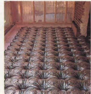
"Airfloor Solar System" is a heat storage/air distribution system, housed in a hollow concrete floor as shown above. Air-floor Systems. Circle 245 on reader service card
