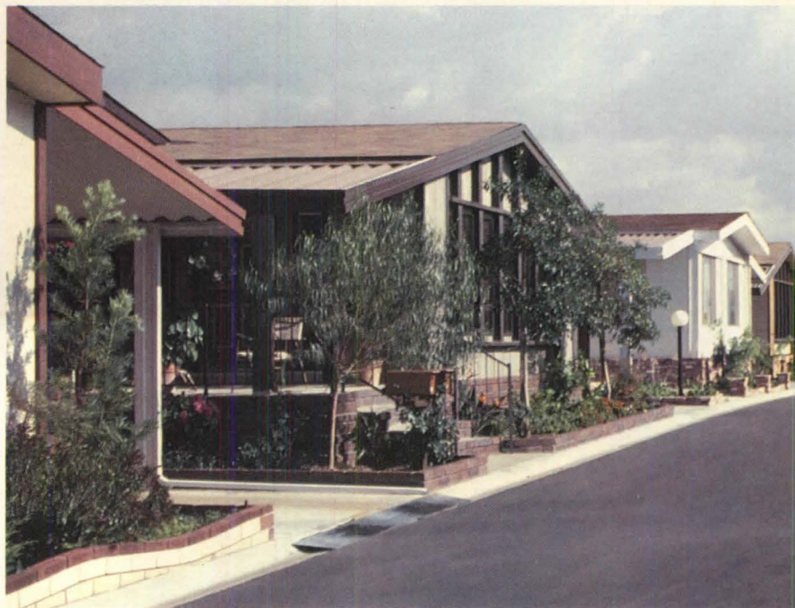
Mobile-home subdivision in Corona, Calif. Units made by Silvercrest Industries.
