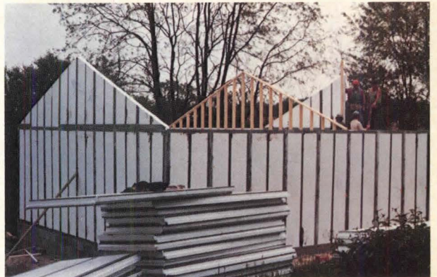
ThermaStructure system is composed of metal bands molded to Structural Expandable Polystyrene panels. In the model home shown above, furring strips are preinserted for drywall installation. No wood studs are used. Radva Plastics. Circle 266 on reader service card
