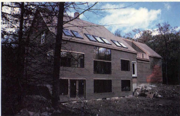
PROJECT: Private home, Walpole, Mass. ARCHITECT: Natural Energy Design, Middletown, R.I. BUILDER: Burke Residential Construction, Walpole, Mass.
