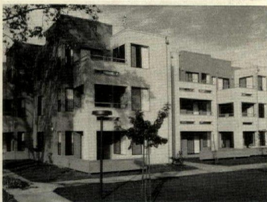
9. Oakland, Calif. Architect: Peters, Clayberg & Caulfield Builder: W&B Constructors
