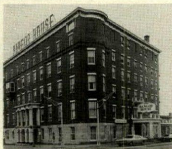
20. Bangor, Me. Architect: CBT/Childs Bertman Tseckares & Casendino Inc. Builder: Myerson/Allen & Co.
