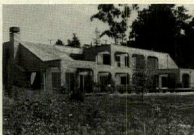
13. Santa Clara County, Calif. Architect: Fisher-Friedman Associates Builder: Vintage Construction Co.
