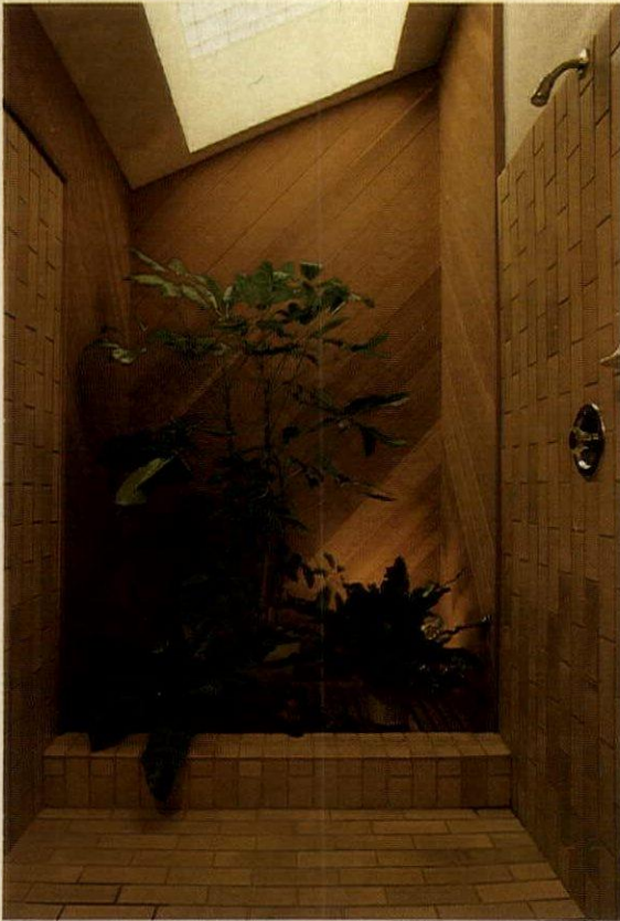
Solar-efficient skylight (above) uses sandwich-type construction with plastic top and bottom to light redwood planter and walk-in shower. Tiled shower has three sets of fixtures, (not shown) including unit "for feet and dogs," in a house by architect Lewis Bishop, Preszler-Bishop, Lodi, Calif. Builder: Leland E. Burns, Woodbridge.
