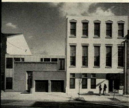
10. Philadelphia, Pa. Architect: Baker Rothschild Horn Blyth Builder: BRHB Developers
