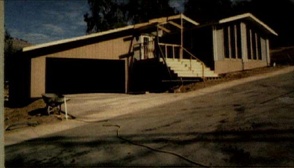
Modular duplex (left) is made from standardized modules shown below. Each unit has two bedrooms and measures 1,152 sq. ft. Homes at Oro Verde, in Escondido Calif. (above) consist of factory-built sections coupled with garages built at the site.
