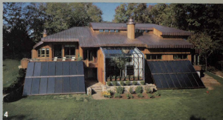
Rear elevation faces south and contains panels for active solar systems plus greenhouse and copper-tube collector for passive system. Notice how the solar panels were integrated into the rear elevation to become an architectural feature. Another advantage: the roof could be designed for esthetics rather than for orientation to the sun. Greenhouse expands visual space in both living room and family room, for its floor was used for thermal storage rather than a thermal storage wall that would have created a barrier.
