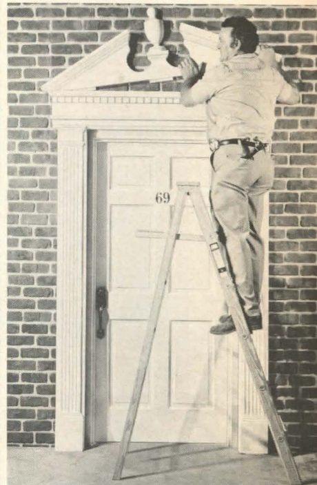
4. Interlock pediment and secure to wall.
