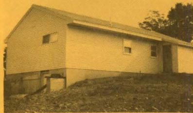
Rear elevation faces north and windows are kept to a minimum. South elevation, on the other hand, has the most window area (see plan above and photo facing page).
