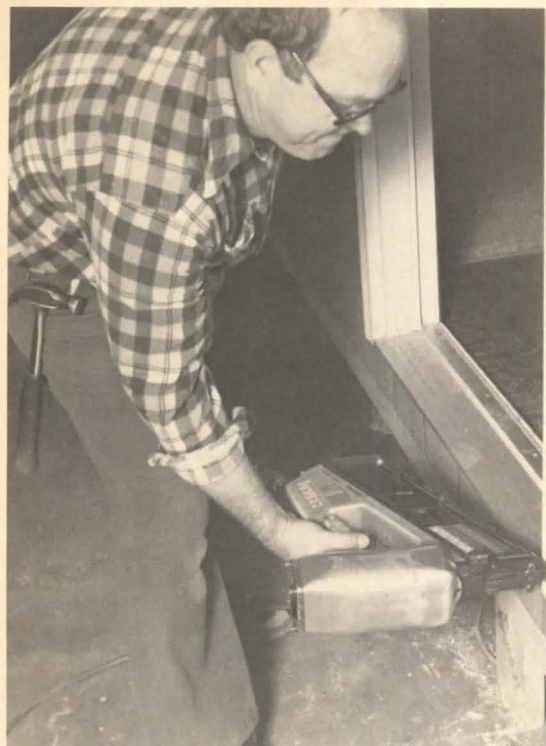
Pneumatic stapler (above) can be used in most applications as a substitute for nailing. Tool is suitable for framing, sheathing and heavy-duty jobs in places that are hard to reach. Senco. Circle 229 on reader service card
