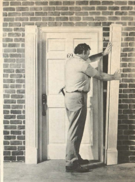
2. Snap pilaster sections onto plates.
