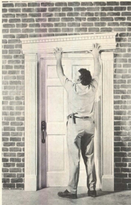
3. Interlock mantel sections and secure to wall.
