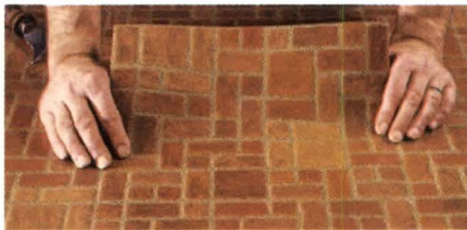
A Tredway patch becomes a permanent part of the overall floor.
