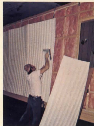
Siding, insulation and caulked seams.
