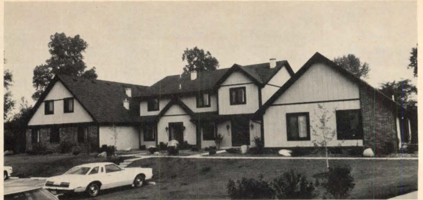
Dug-out parking (above) hides cars from tenants' view. Earth was moved to form mounds that shield side patios. Cost: $5,000 per building.
