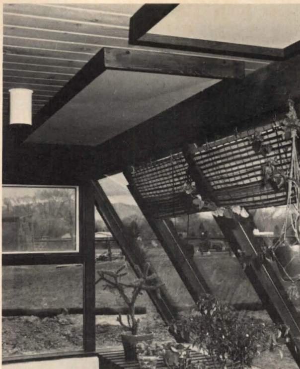
Electric radiant heating panels (above) are suitable for use in greenhouse-type extensions. The surface-mount ceiling units range from 2' x 2' to 2' x 8' in size and from 375 to 1500 watts. Aztech, Albuquerque, NM. Circle 236 on reader service card
