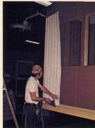
Siding, insulation and Fome-Cor sheathing board.
