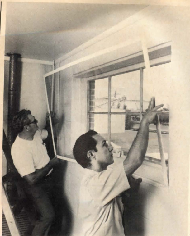
Heavy-duty interior storm window (above) is designed for commercial and apartment applications. Window is made of clear acrylic and comes in standard and custom sizes. Plaskolite, Columbus, OH. Circle 227 on reader service card
