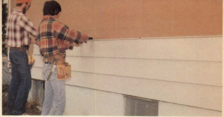
"Firm, even walls make residing jobs go fast!"
