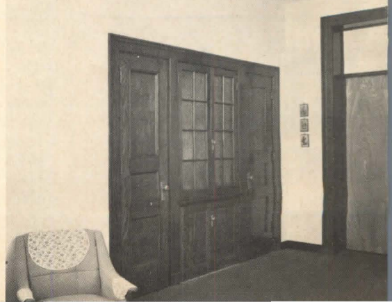
Classroom closet at Central Grammar School is still in use in a tenant's living room. The old door, however, had to give way to progress.
