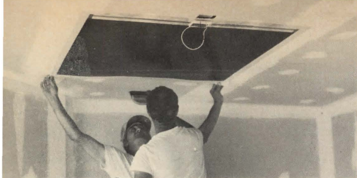
3. Installation: Aligned panel is bonded to ceiling.
