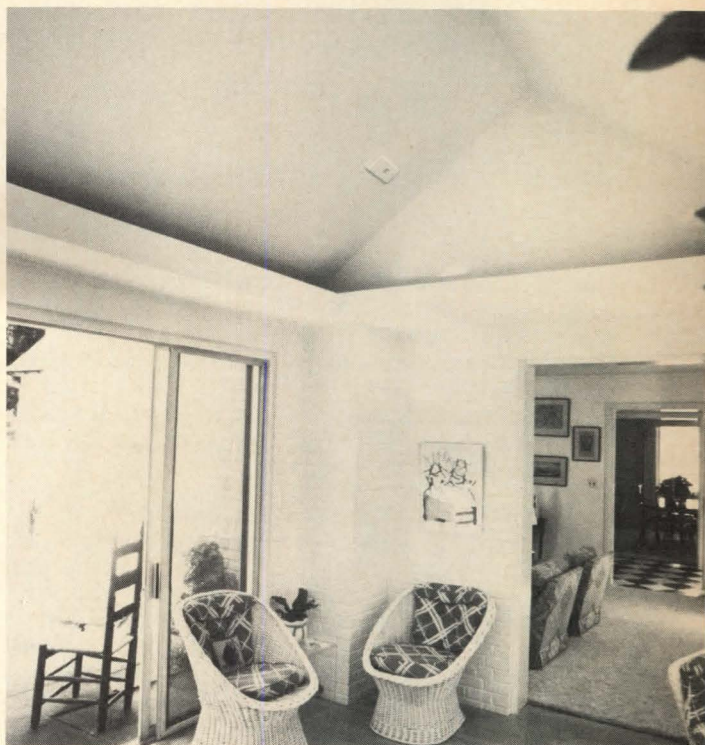
Finished application: Heating panel blends into rest of ceiling when painted over, as shown above. Only junction box is visible.
