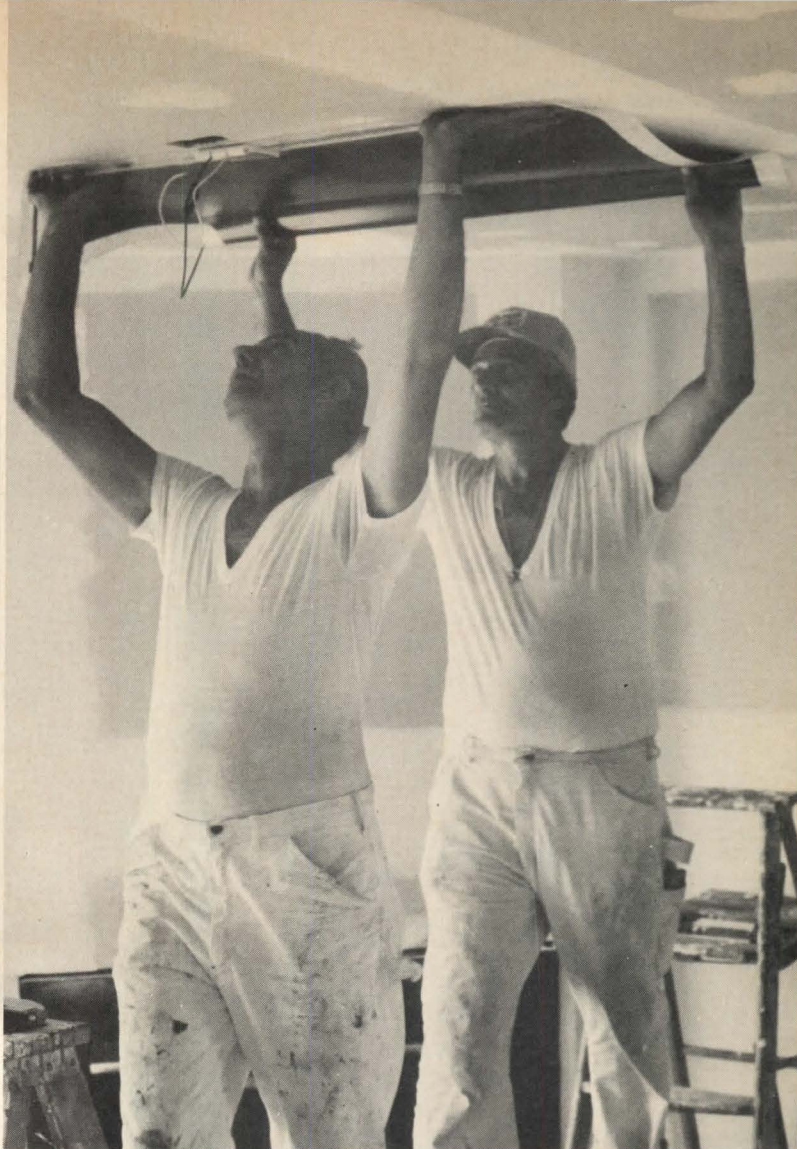
2. Alignment: Panel is readied for positioning.
