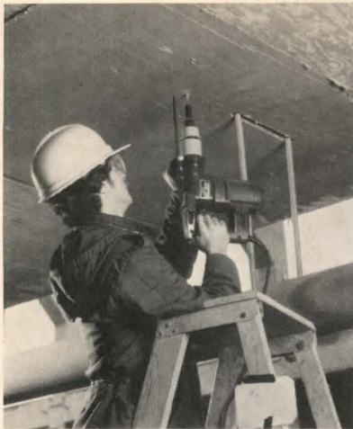
Electro-pneumatic rotary hammer , "Mars 717" (above), delivers 3,150 blows and 550 rpm. Lightweight tool weighs 10½ lbs., and requires only 10 lbs. of contact pressure. Rear handle shape allows greater room for the operator's hand. A switch controls speed and operation. Skil, Chicago. Circle 208 on reader service card
