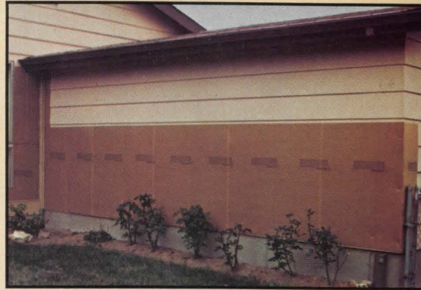
Fome-Cor board wraps homes like a blanket. Folds around corners. Cuts with a knife.
