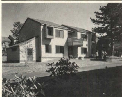
25. Winthrop, Mass. Architect: Goody, Clancy & Associates Inc. Builder: Bick-Com Corp.
