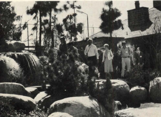
Crossing bridge at Quail Ridge, builders admire waterscaping.
