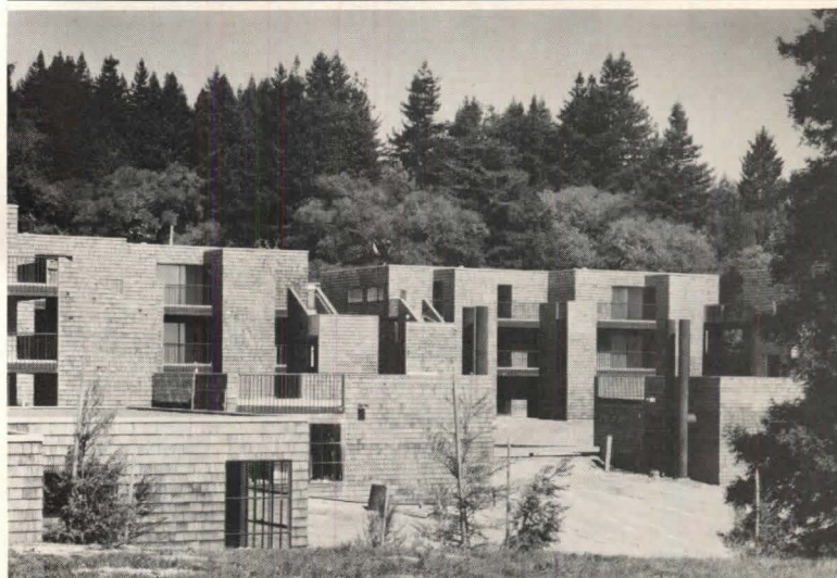
1. Santa Cruz, Calif. Architect: MBT Associates Builder: Williams & Burrows
