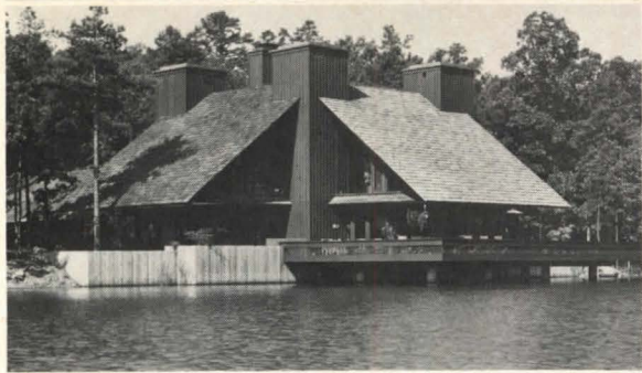
18. Little Rock, Ark. (vicinity) Architect: E. Fay Jones Builder: Herb Davis
