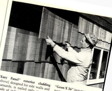
"Easy Panel" (above), designed for side walls and mansards, is nailed only at studs. Made of individual #1 Centigrade Western Red Cedar shakes and shingles bonded to a 4'-long wood backing, panels come in five textures including roughsawn shown. Shakertown Panels, Winlock, Wash. CIRCLE 224 ON READER SERVICE CARD
