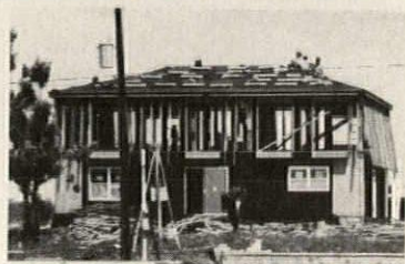
New home rises in Pinecrest, where $40,000-$50,000 units were leveled.
