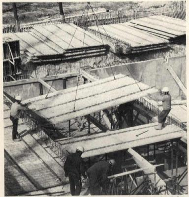
Semi-precast slab system, "Dawide", is for fire-resistant roof and floor construction. A thin portion of a concrete slab is precast in factory and reinforced by a protruding light steel truss and steel mesh. Slab is completed on site by pouring another layer of concrete. The smooth underside serves as the ceiling and the top of the slab accepts flooring or roofing materials. Bowsteel, Linden, N.J. CIRCLE 214 ON READER SERVICE CARD
