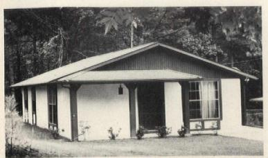
Simple structural system, shown in a completed house, consists of building blocks and a mortarless surface bonding cement, Surewall<sup>®</sup>. The blocks are stacked in a running pattern; then the bonding cement is mixed and troweled onto the sides providing a smooth, white, moisture resistant finish. W. C. Bonsal, Lilesville, N.C. CIRCLE 212 ON READER SERVICE CARD
