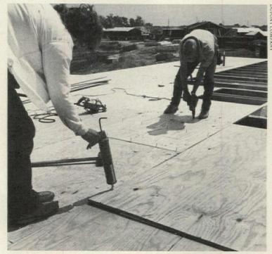
Adhesive is applied to plywood subfloor edges (foreground), while worker at rear secures subfloor to steel C-beams with self-drilling screws.
