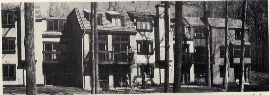
Rear townhouse balconies are staggered to provide greater privacy between units. Townhouse floorplans (below), which range from 2,130 to 2,470 sq. ft., show how units are arranged within a typical
