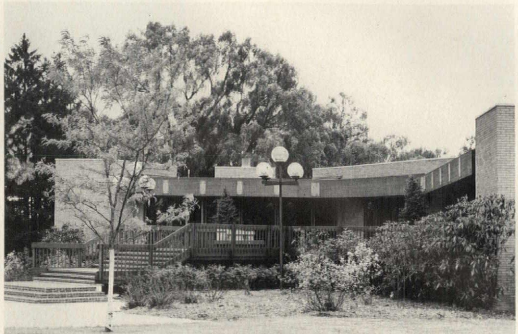
Recreation building, with indoor and outdoor swimming pools, was planned for 4,000 families and cost $700,000. Today there are only 400 families living at Greenwood and using these luxurious amenities.
