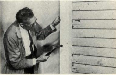
2. Corner posts. Place posts on all inside and outside corners, allowing 1/4" at the top. Position the post by placing nail at top of upper slot, placing all other nails in the center of the slots.
