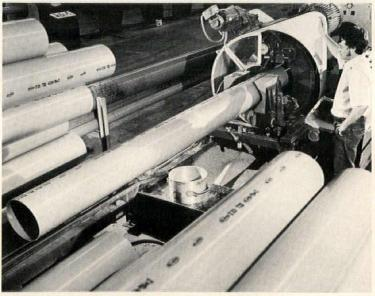
Water transmission pipes, manufactured of Goodyear PVC plastic, utilize a patented Bell-tite joint system that eliminates the need for cementing or solvent welding. The system permanently seals two lengths of pipes using a rubber gasket. Plastic pipes-12" in diameter or less-can also be adapted to iron pipe jointing systems to permit a smooth transition from iron to plastic piping. Clow, Pell City, Ala. CIRCLE 243 ON READER SERVICE CARD
