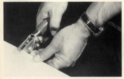
**9. Last panel.** Cut it to cover the remaining open section. Punch lugs every 16"-24" along the cut edge with snaplock punch, raising lugs on outside. Then lock siding into the undersill trim placed under the eaves.
