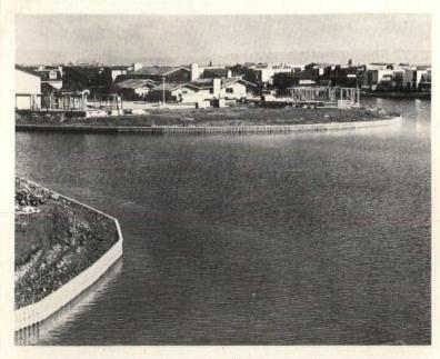
Marine retaining-wall system, Shore All<sup>TM</sup> protects waterfront property from the sea. A special corrosion-resistant corrugated bulkhead is formed from sheets of durable aluminum. Sheets are joined by sand-tight ball-and-socket joints and capped with an aluminum alloy extrusion that is bolted into predrilled holes. Kaiser, Oakland, Calif. CIRCLE 231 ON READER SERVICE CARD
