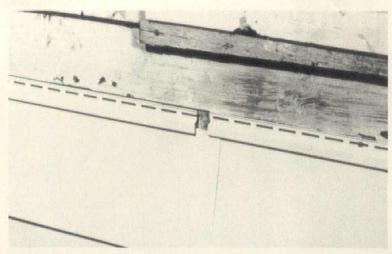
**6. Lapping panels.** Lap siding half the length of the prenotched ends. Stagger laps so one is not above another, unless separated by 3 courses, checking every 5th or 6th course for alignment. Always overlap joints away from entrances and traffic flow to improve appearance.
