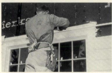
8. Fitting around window. Nail J channels on window and door sides and tops, and undersill trim on window bottoms, to receive siding. (Vinyl window head flashing should be used above doors and windows unless previously flashed.)
