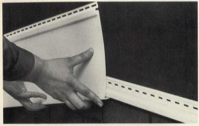
**5. First panel.** Lock it into the starter strip, placing backerboard behind. Leave ½" at all corner posts and channels. If individual corner caps are used, cut back panels ½" from corner.
