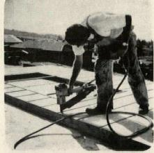
Fast on-site component construction with CN-137
