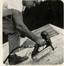
Staple Natier anchors down plywood roof deck
