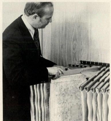
Vertical filing system for blue prints and plans features self-centering pivoted binders that clamp up to 100 sheets without pre-fastening or punching. The 18"-wide modular racks can be wall mounted as shown or used as mobile files. Rigid steel brackets with stud mountings provide secure suspension for file. Plan File, Los Angeles, Calif. CIRCLE 297 ON READER SERVICE CARD
