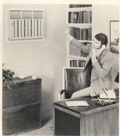
Through-the-wall air conditioner has a high efficiency rating to hold down operating costs and conserve electricity. Unit, with a slide-out chassis for easy installation and service, features a temperature-anticipating thermostat, a six-way air control, an oversized condenser coil and an anti-ice device. Freidrich, San Antonio, Tex. CIRCLE 243 ON READER SERVICE CARD
