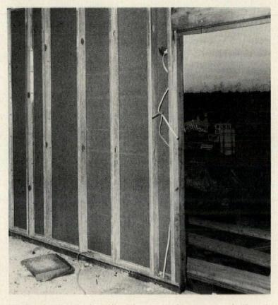
Metal stud system, for dry wall or plaster, provides extra strength. The web of the stud is reinforced with both horizontal and vertical ribs. Constructed of several gauges of steel, the easy-to-install units can be cut to fit. Warpand flameproof studs in a variety of sizes accept screws or glue. Vulcan, Birmingham, Ala. CIRCLE 225 ON READER SERVICE CARD
