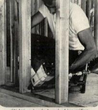
CN-137 makes fast work of loe-nailing
