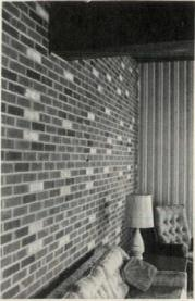
Easy-to-install thin bricks for interior application are the same height and width as traditional bricks but are only ½" thick. Brick wall is applied by spreading a layer of mastic on the surface to be covered and pressing the Brickettes® into place. Available in 12 color blends. Modern Methods, Evansville, Ind.
