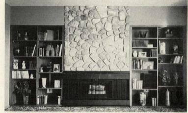
Simulated stones fabricated of plastic are made to look and feel genuine. The stones, available in three colors—natural, gray and white—have a rough texture like that of real stone. No two surfaces are exactly alike. Easy-to-install stones are pressed onto a mortarlike adhesive background. Design Images, Manchester, N.H. CIRCLE 231 ON READER SERVICE CARD
