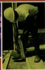
A new weight-saving power source design with wafer piston makes the SKO-35 the most powerful tool on the market, pound for pound. It drives nails home in hardest woods.
