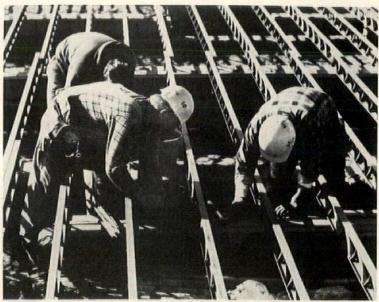
**Lightweight steel truss** is part of a structural system that also includes a header channel and load clip. Suitable for roofs, floors, load-bearing and chase walls, the truss features an open web design. It is available in sizes 2'x6' and 2'x8' (to compete with wood joists) and in lengths to 50'. C/O, Detroit, Mich. CIRCLE 209 ON READER SERVICE CARD
