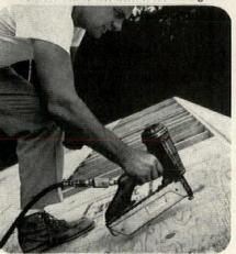
Staple Nailer anchors down plywood roof deck
