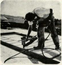
Fast on-site component construction with CN-137
