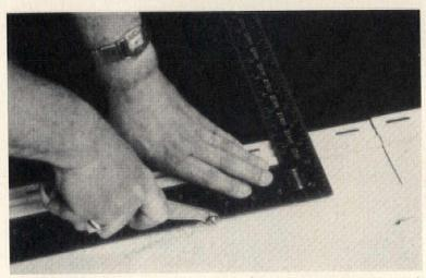
7. Cutting for windows. Mark the section to be removed, cutting the sides with snips and scoring lengthwise with a utility knife or scoring tool. Bend the section along the scored line to remove.
