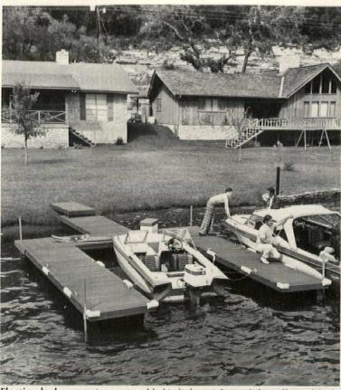
Floating dock system is preassembled in lightweight modules. All wood deck components are impregnated with a preservative. Deckboards are finger-jointed with waterproof adhesives and notched to prevent cupping. Sideboards are laminated for strength. Flotation is provided by non-sinkable polystyrene foam. Koppers, Pittsburgh, Pa. CIRCLE 201 ON READER SERVICE CARD
