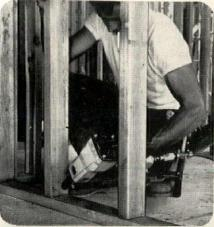
CN-137 makes fast work of toe-nailing
