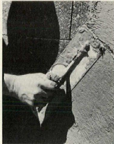
Glass-fiber bonding material eliminates the need for mortar in concrete-block construction. "Bloc-bond", in 80 lb. bags, is a mixture of Portland Cement, hydrated lime, a water-resistant agent and alkali-resistant glass fibers. The easy four-step application process is shown above. Owens/Corning, Toledo, Ohio. CIRCLE 208 ON READER SERVICE CARD
