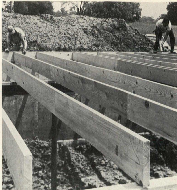
End-glued dimension lumber, meeting federal standards and code specifications, is available kiln-dried in lengths up to 40' in 1/8" increments. Suitable for use as joists or truss chords, the long lumber has fine tolerance finger joints bonded with fully waterproof adhesives. Weyerhaeuser, Tacoma, Wash. CIRCLE 207 ON READER SERVICE CARD
