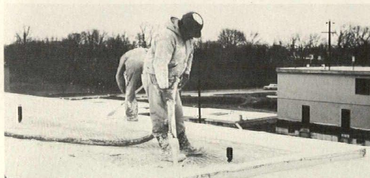
Roof deck system, familiar in non-residential construction, can now be used for wood-framed garden apartments. "Pyrofill" or "Thermofill" gypsum concrete slabs satisfy fire codes without above-deck firewall extensions and also allow drainage slopes to be formed on the roof. U.S. Gypsum, Chicago. CIRCLE 205 ON READER SERVICE CARD
