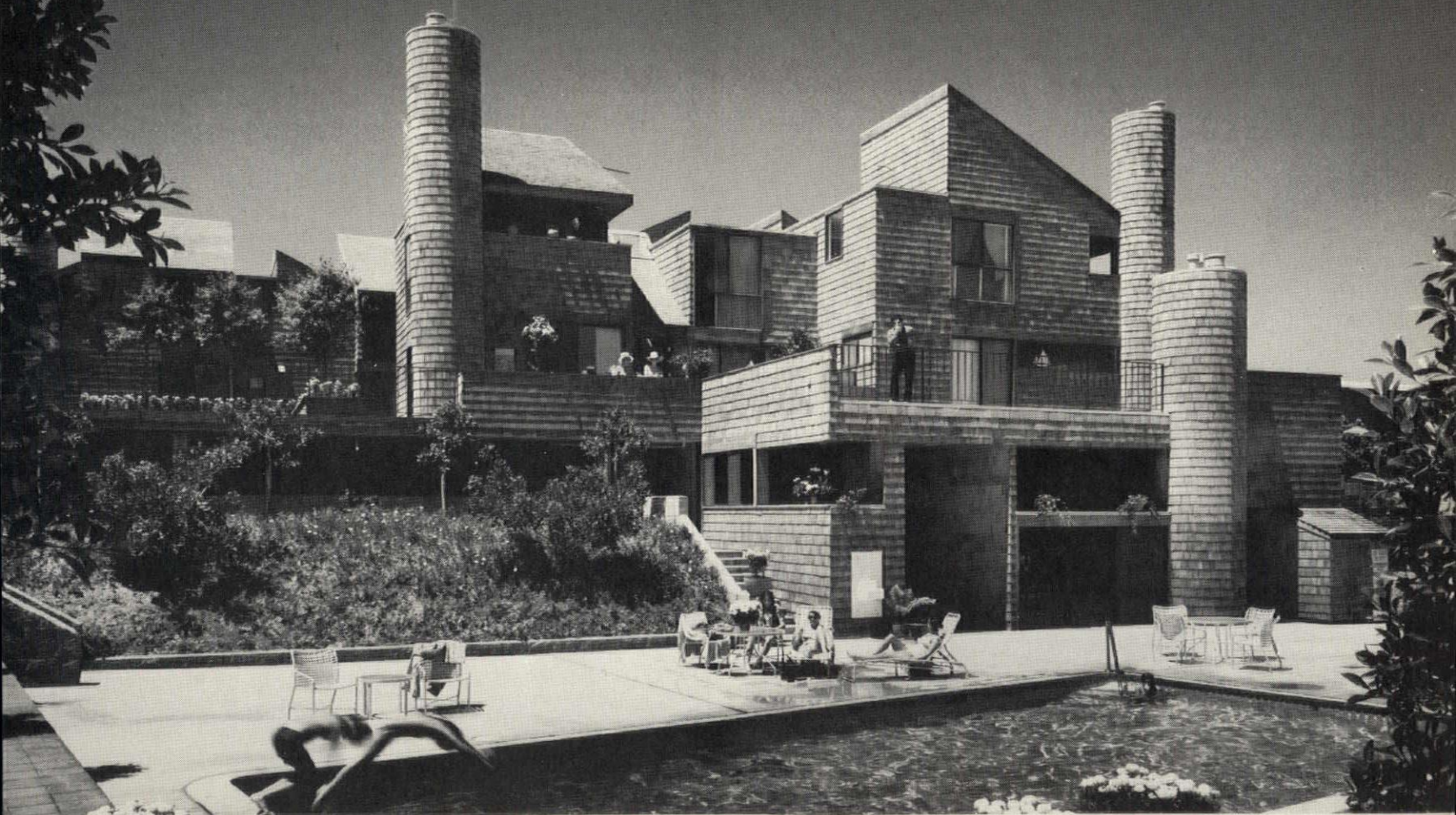
Seascape I, Solana Beach, California. Roofs: Certigrade shingles No. 1 Grade, 24" Royals. Walls: Certigrade shingles No. 1 Grade, 16" Fivex. Architects: Oxley & Landau. Builder: Westward Construction Corp.
