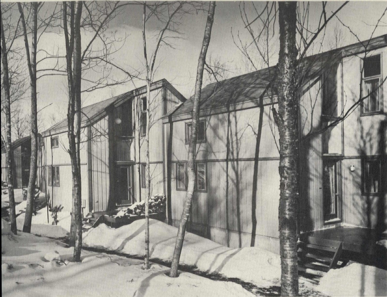
Panelized building (above), one of several styles supplied by Acorn Structures, contains layouts shown on opposite page. Main ski area (left) includes the base lodge and multi-level units over two floors of commercial space—a restaurant, ski shop, laundry, photo shop and country store. Architect for this stick-built structure was Ecodesign.
