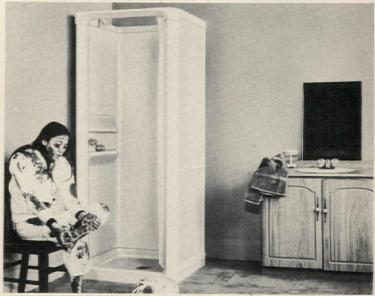
Shower cabinet, thermo-formed of modified acrylic, is non-rusting, stain resistant and never needs refinishing. Unit comes complete with factory-installed drain and
