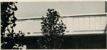
Facade panel system, for singlefamily or high-rise construction, will not rust or corrode and has a Class I fire retardant rating. Vertical tracks, mounted on a structure, support PPG fiber glass reinforced pan-
