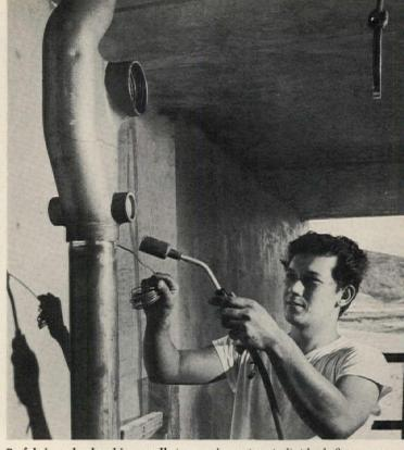
Prefabricated plumbing wall is a self-aerated one-stack drainage system suitable for two-story garden apartments to 40-story office towers. Savings of up to 12 feet of water tubing can be achieved per bathroom by using individual fixture stops. In a back-to-back bath arrangement, one lightweight set of hot and cold lines can do the work of two. Copper Development, New York City.
