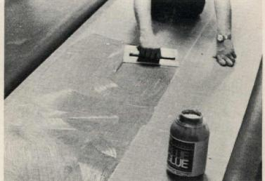
Carpet adhesive has coverage of 80 sq. yds. per gal., about 7 times the normal, which results in greatly reduced installation costs. Suitable
