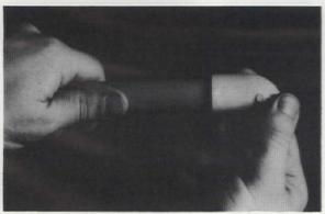
Push the tubing into the fitting. Then give either the tubing or the fitting a quarter turn to insure proper distribution of cement. Immediately adjust for direction. Wipe excess cement from the fitting lip; hold both together for a few seconds.
