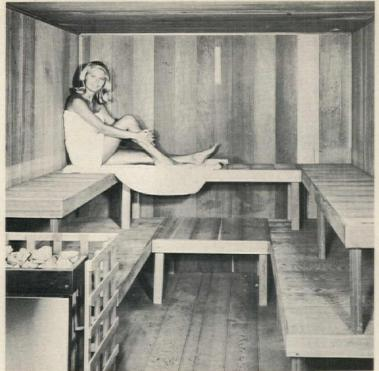
Jumbo saunas with 80 sq. ft. of floor space can accommodate 15 people sitting down. Interior walls, ceilings, floors, benches and heater fence are constructed of kiln-dried redwood. Exterior is laminated fir plywood. A polyurethane foam bond between the exterior and interior
