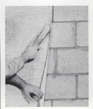
A fire-resistant roll of plaster in a scotch weave is used in the same way as conventional wallcoverings. Offered in 48"-wide rolls, the surfacing material can be directly applied with an adhesive to any rigid surface including concrete block. The covering remains flexible until it is applied at which time water in the adhesive sets the plaster. Flexi-Wall Systems, Liberty, S.C.
