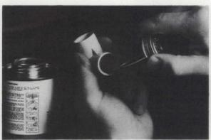
Remove surface gloss from the tubing end and fitting socket with CPVC cleaner or fine sandpaper and wipe clean with a dry cloth. Brush CPVC cement to the inside of the socket.
