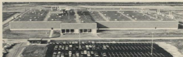
New 275,000 sq. ft. Building Products manufacturing facility, Ashville, Ohio.
