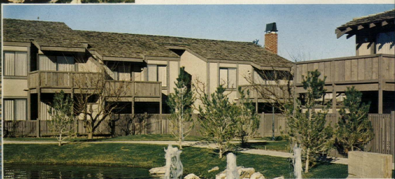
Glenbrook Garden Apartments. Architect: Donald Sandy, Jr. A.I.A. and Anthony Guzzardo A.S.L.A. Builder: Avery Construction Co.
