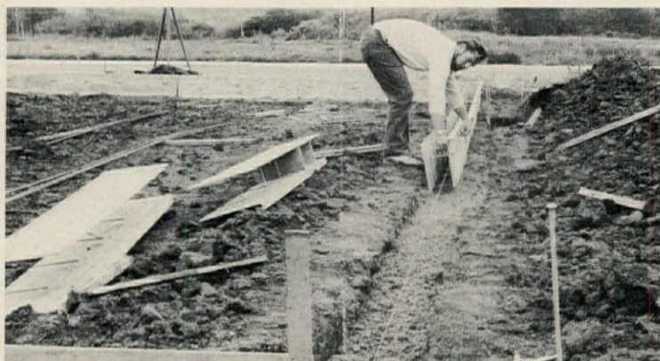
Modular foundation-forming system for slab houses uses no stakes, yokes or braces. Modules are fabricated of outside and inside panels, held together with steel cross ties to resist pressure of the concrete. Lightweight modules can be re-
