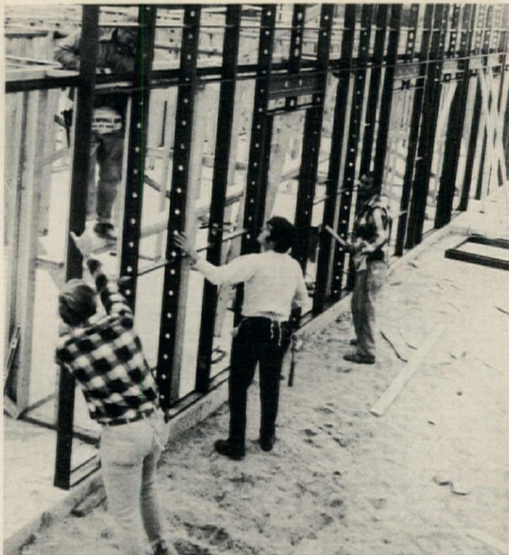
Structural steel panel system for light construction replaces individual studs welded on the job. Load-bearing system is factory assembled, eliminating waste and theft of material for the builder.
