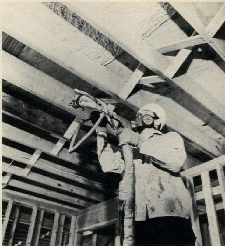
Rigid polyurethane foam system can be used structurally as well as for insulation. Sprayed to the underside of a floor (shown), the foam insulates, strengthens and reduces vibration. As a wall composite, it
