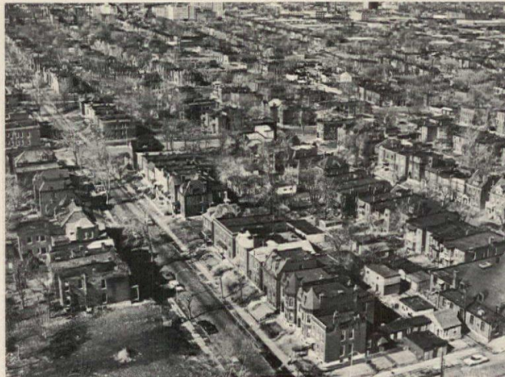
Abandoned and vandalized, FHA-subsidized homes stretch through center of St. Louis. Survey found one fourth were occupied less than a year before foreclosure. "I wish I was back at Pruitt-Igoe," said a welfare mother who bought house, only to have it crumble. She referred to the public housing now being partly demolished by HUD.
