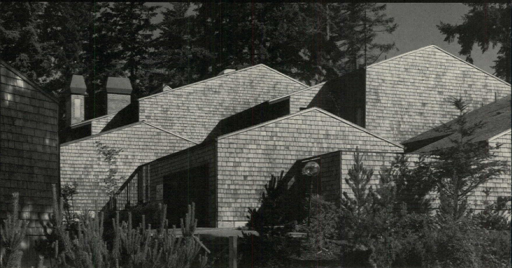
Condominiums, Mountain Park, Oregon. Certigrade Shingles No. 1 Grade: roof, 18" Perfections; walls, 16" Fivex. Architects: Broome, Selig & Oringdulph.
