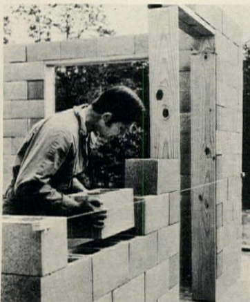
Modular foundation-forming system for slab houses uses no stakes, yokes or braces. Modules are fabricated of outside and inside panels, held together with steel cross ties to resist pressure of the concrete. Lightweight modules can be re-
