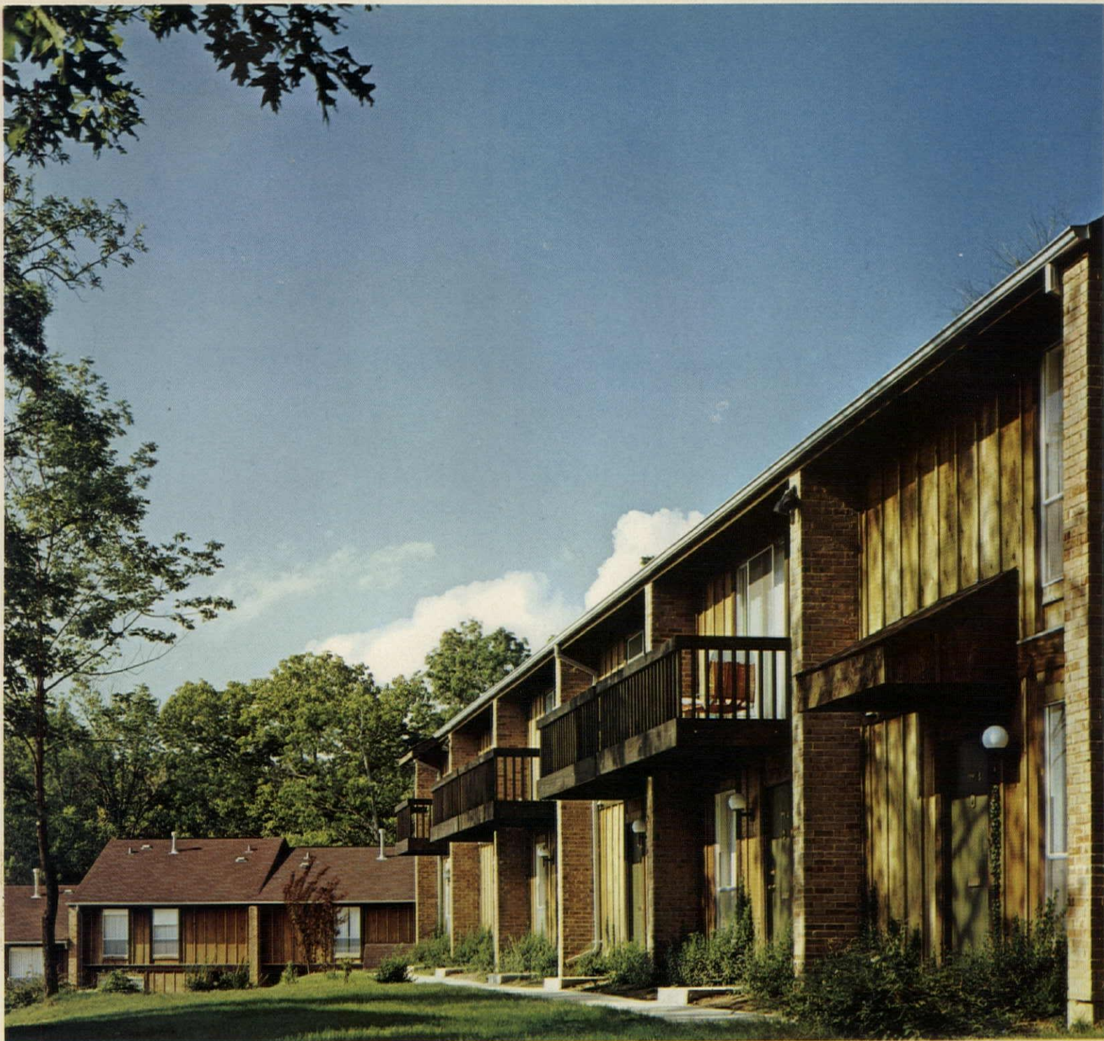
Charter Oak Townhouse and Apartment complex, St. Louis, Missouri, features use of Non-Com® Exterior for board and batten cedar siding. Developer: Lincoln Property Company, St. Louis. Architects: Dale E. Selzer, AIA, Dallas; Hastings and Chivetta, AIA, St. Louis.
