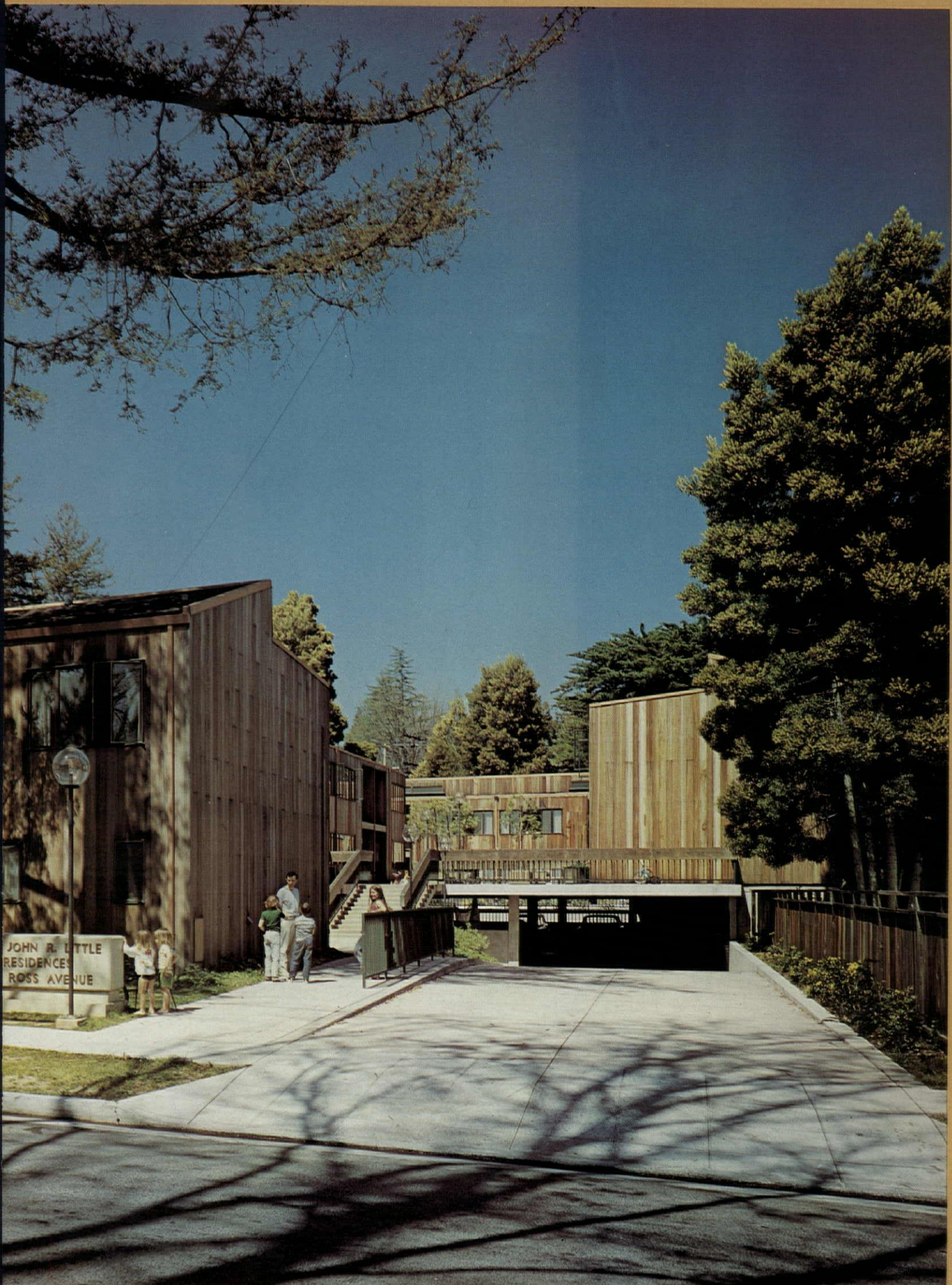
Below-grade parking saves space on a small site in San Anselmo, Calif. For a closer look at the project, turn the page.
