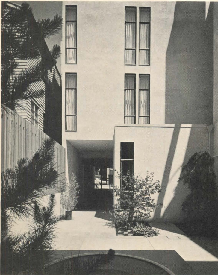
Side courtyard, seen from recreation room (see ground level plan, right) provides a view for six units. It leads to street entrance (background, photo, above).
