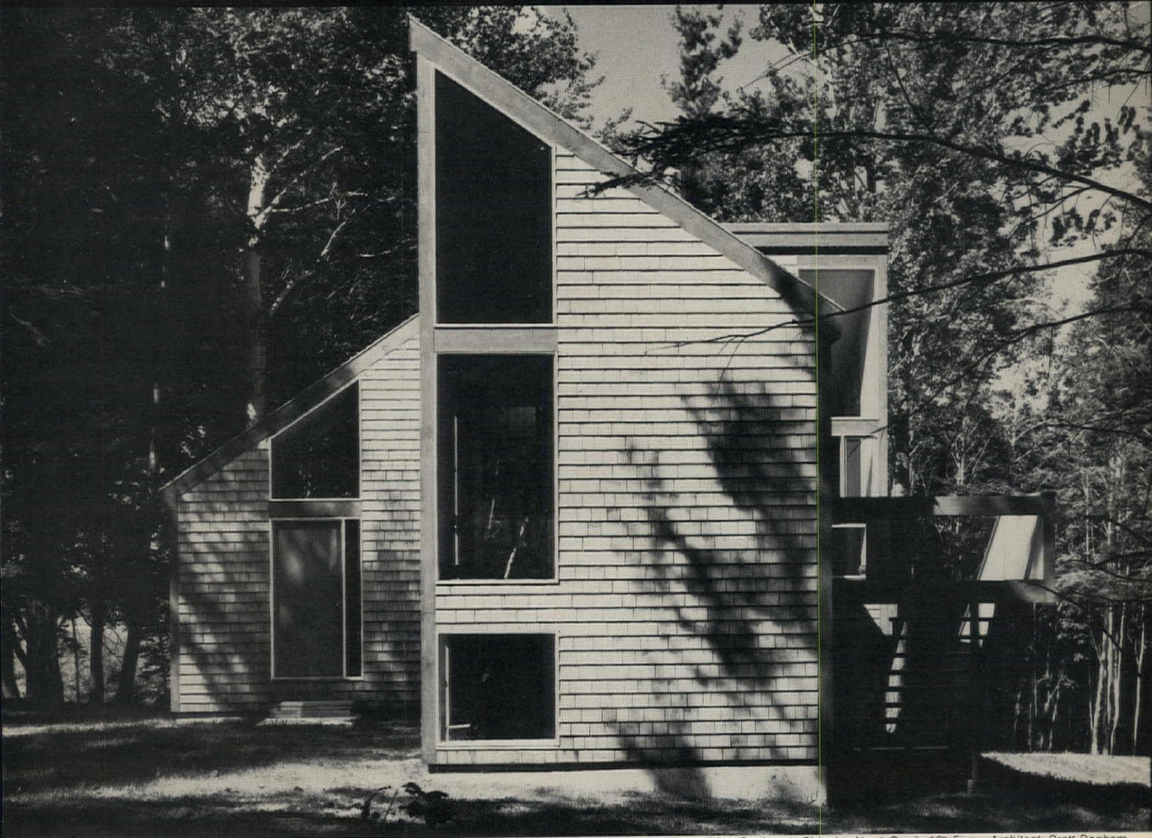
Vacation home at Franconstown, New Hampshire. Certigrade Shingles No. 1 Grade 16" Fivex. Architect: Brett Donham.
