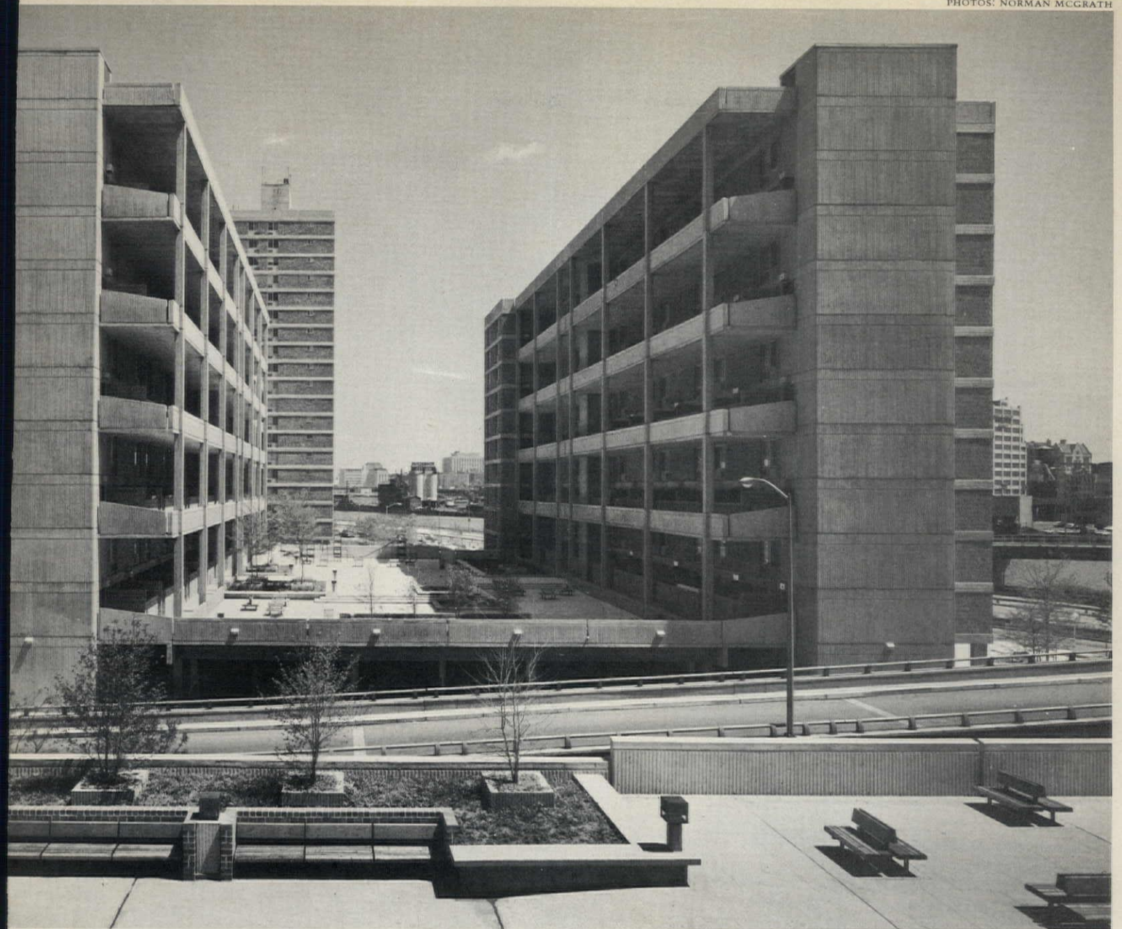
Riverbend Housing's site is bisected by a ramped approach to the Harlem River Drive (photo, above and plan, opposite page). To tie the two areas together visually, courts were erected, at the ramp's level, between buildings on either side of the ramp; they seem to bridge the roadway. Floor plans below are of duplex apartments in the low-rise buildings.
