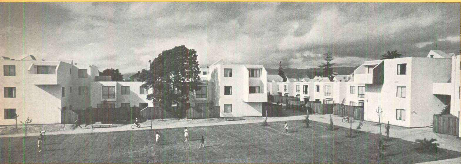
Wood frame buildings in project have double-stud walls and stucco exteriors. Three-story corner units are shown above.
