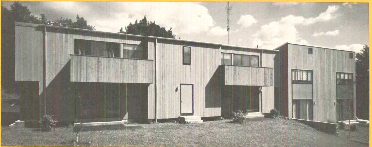
Efficiency apartments in this building have balconies and basements. Retaining wall divides one-bedroom from two-bedroom units.
