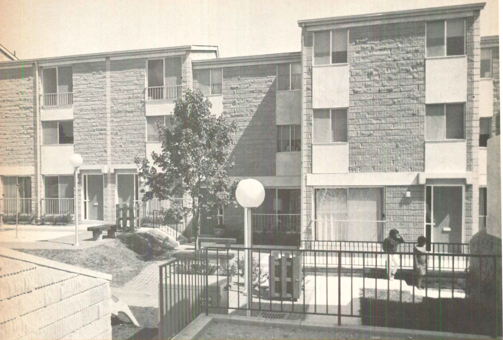
Corduroy brick and precast concrete panels are low maintenance materials used for exteriors. Buildings are air-conditioned.
