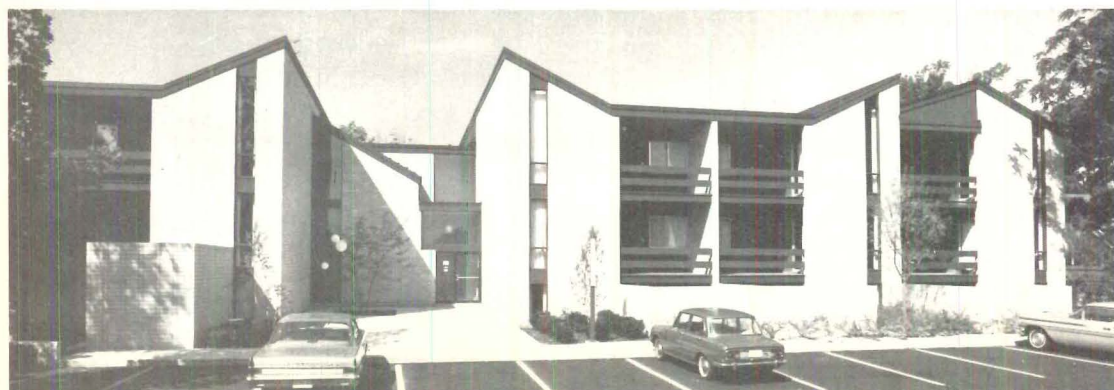
Apartment building on rear of lot was completely rented within two months after completion. Both buildings are of lightweight concrete brick.
