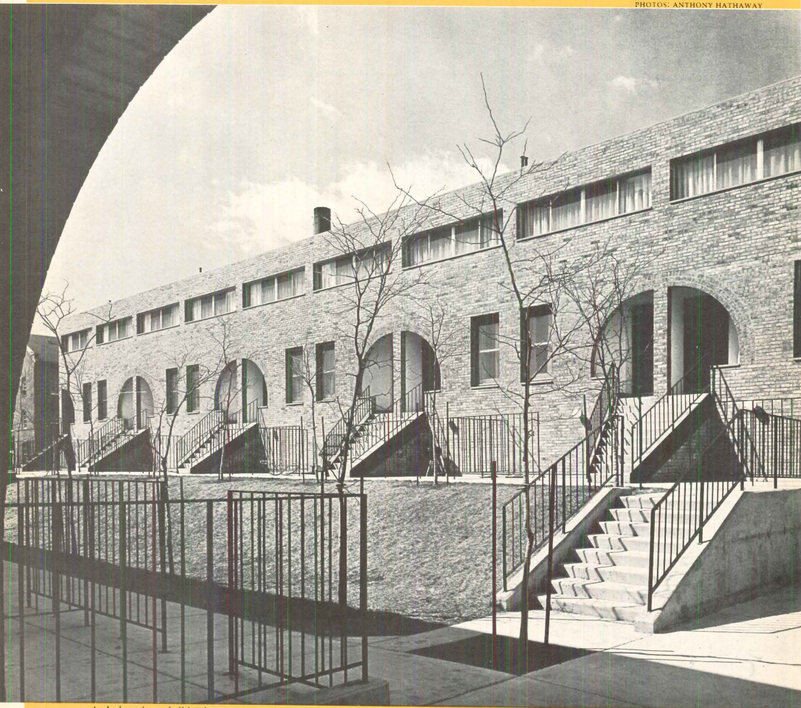
Arched entries and all-brick construction characterize Channel Square project. This is last land parcel in area to be put up for redevelopment.
