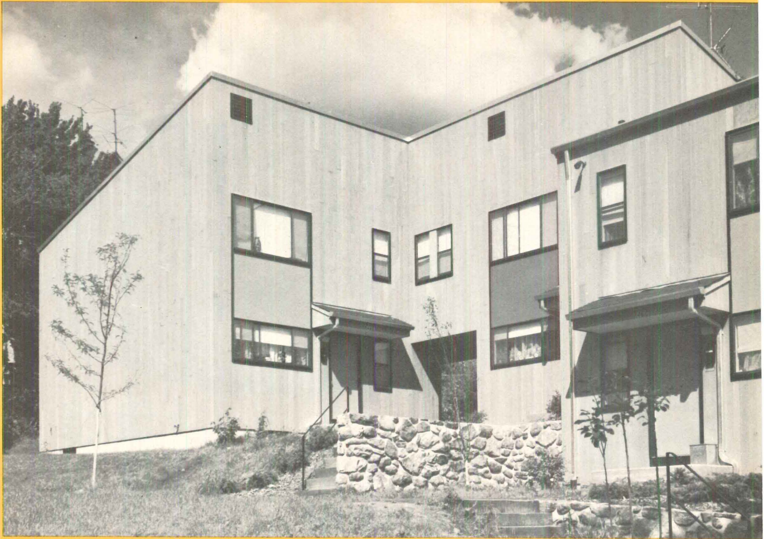
Stepped-down design (see also site plan, facing page) has series of retaining walls and offsets to conform to sloping terrain.
