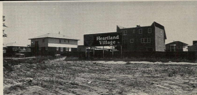
Street sign (above) for typical 100-150-unit Staten Island project has size to commend it, but it can't match the lush setting of the entrance sign to Village Greens (right). Set on a wall and gate post of the same stone used on its buildings, the sign at the main entrance of Village Greens greets visitors with distinctive lower-case typography. The square symbol at lower right of sign is repeated on all promotion material.
