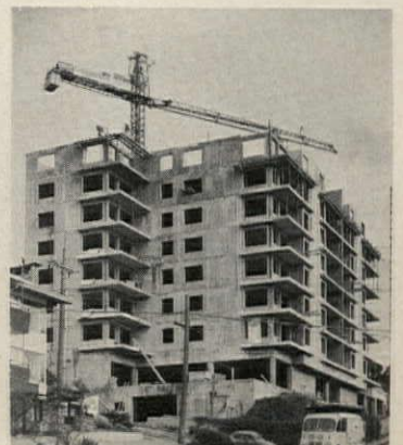
Continental House is first of two projects to use precast panels.
