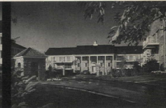
1968: Toledo's largest project—462 units
