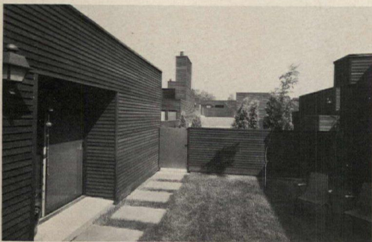
Private courtyard in each unit is 18' x 24'. End wall allows view out, but retains owner privacy—it is 4½' high inside, 6' high outside (photo, above).
