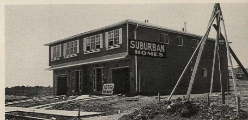
Sales office for typical Staten Island project (above) is in a model home. In sharp contrast is the handsome Village Greens' sales pavilion (right), with continuous strip of windows and rear deck overlooking the models. Grass was well established when the project was opened, and landscaping was completed. Every effort was made to retain all trees; those that had to be moved were replanted elsewhere. Parking area is beyond the picket fence at right.
